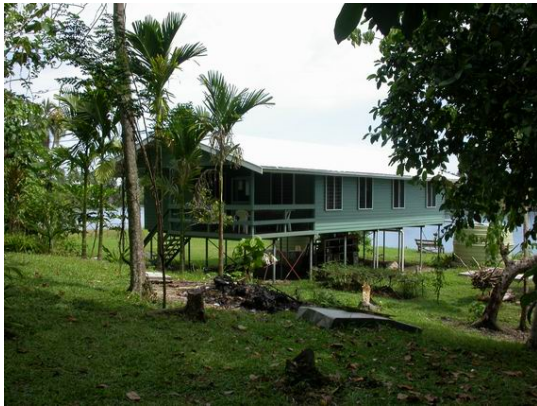
Fig 4. New Darwin-funded dormitory building
